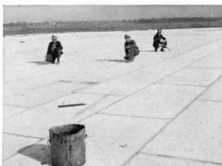
Caulking joints between Cemesto panels. Carolina Asbestos Co., Marshville, N. C. Contractor: Interstate Const. Co. Architect: A. G. Ulrey.
