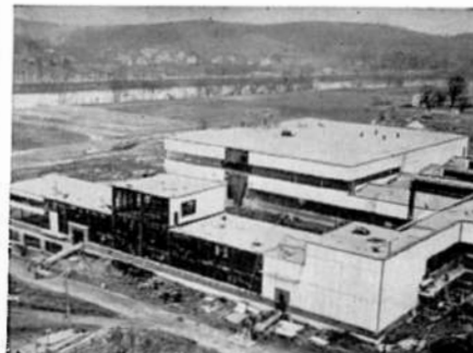
42,000 square feet of Cemesto used for roof deck and curtain walls. B. F. Goodrich Co., Marietta, O.
