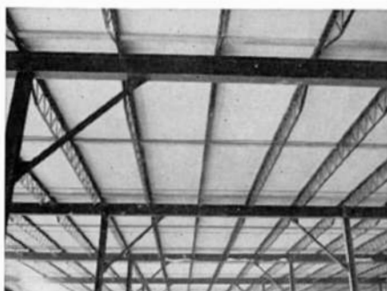
Light steel framing for 53,760 sq. ft. of Cemesto for Watson Terminal Warehouse Company, Youngstown, Ohio.
