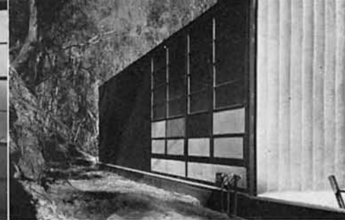
Exterior of the same sash shown at left. The vertical Ferroboard shown here on the court side is painted aluminum.
