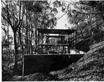
IT BECOMES AN AIRY PAVILION WHEN THE FERROBOARD ROOF DECK IS APPLIED.
