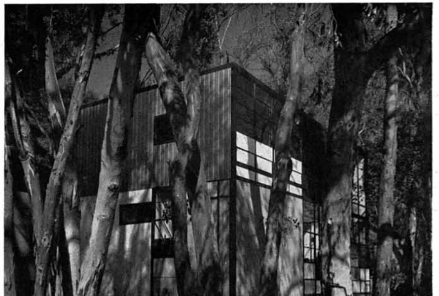
All steel sections, metal sash and flashing are painted a dark neutral gray, which enclose the buildings in a sharply defined structural web.
