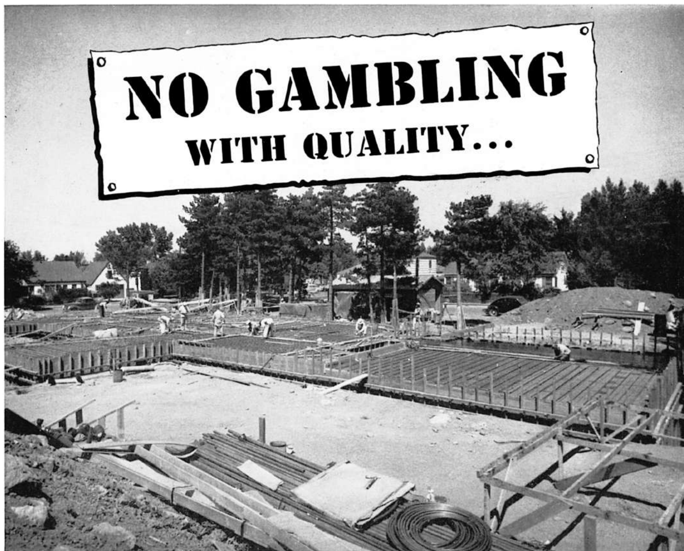
11,000 feet of Revere Copper Water Tube were used in the radiant panel heating system. The building has 9 zones, with each room controlled by individual thermostats. Revere Copper Water Tube was also used for hot and cold water lines, and Revere Sheet Copper for roofing.
