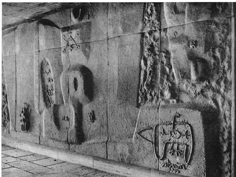
The base of the 30-foot high bas relief; made of reinforced concrete, cast in sand molds, the bas relief, 16 feet wide, rises 30 feet beside a stairwell in the main dining room. The section pictured is 8 feet high.
