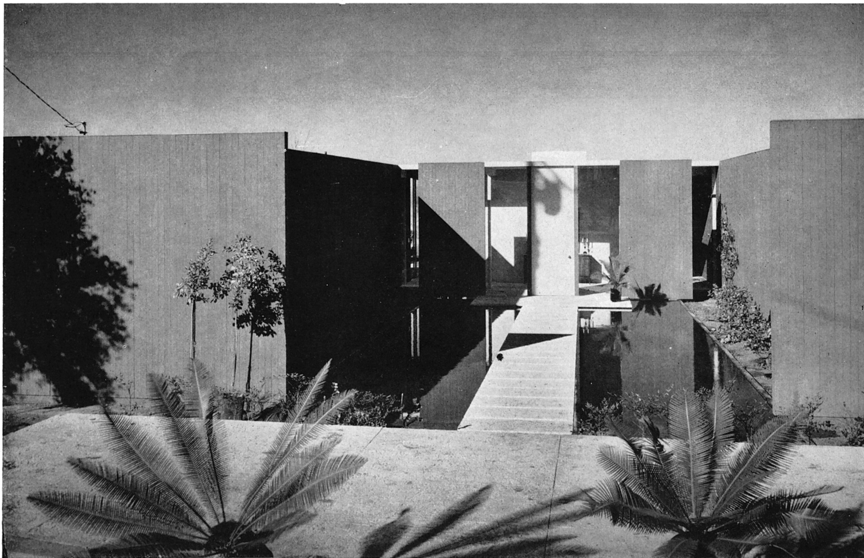
Entry court showing the white pre-cast stepping stones leading across the shallow reflecting pool to the 10'-high entrance door. The handsome exterior walls are of butt joint T & G resawn redwood finished with Pittsburgh Paints' Rez stain.
