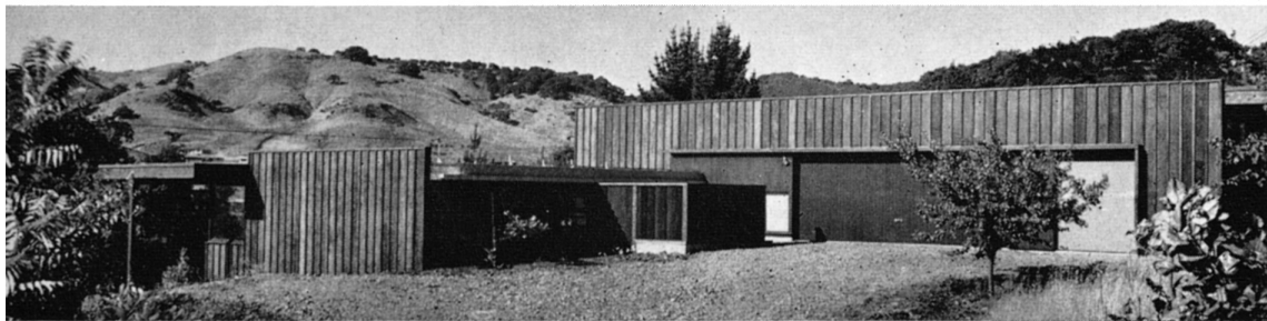
GARAGE AND SERVICE ENTRANCE
