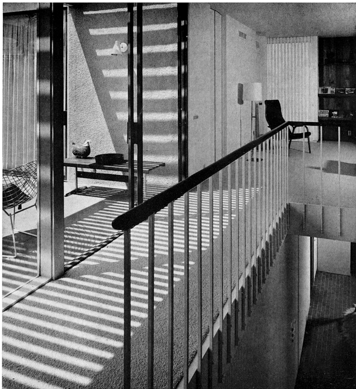
The stair rail is of wrought-iron with a shaped walnut handrail. Terrace to the left, study in the background. The dining room is below. The Swepe lighting controls are simply located at a 3'-0" height on all the walls.
