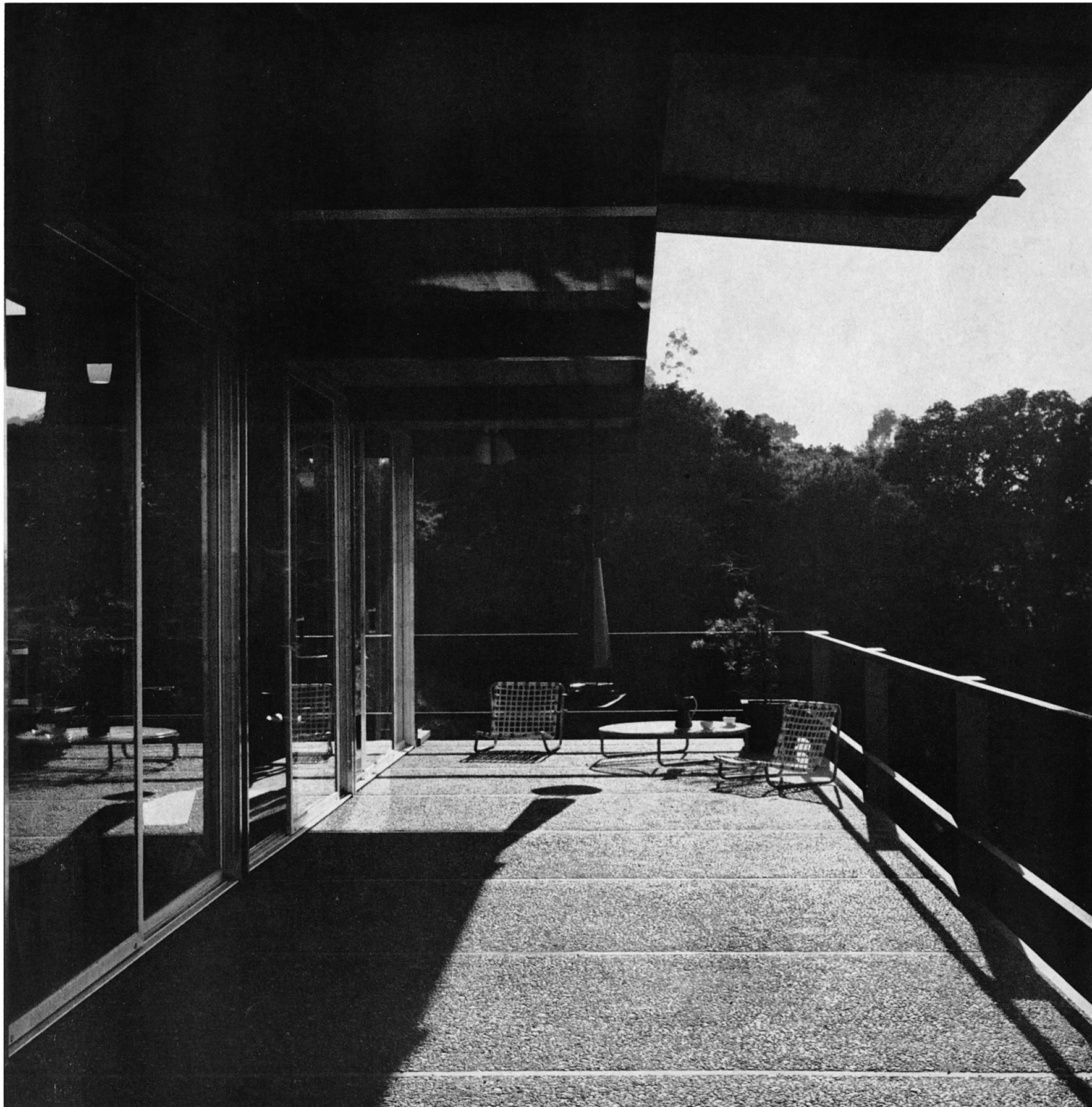
The 10-foot-wide cantilevered deck, overlooking the golf course and the hills beyond, provides 800 square feet of deck, most of it covered. The finish over the exposed concrete aggregate is "Holztite" concrete sealer.
