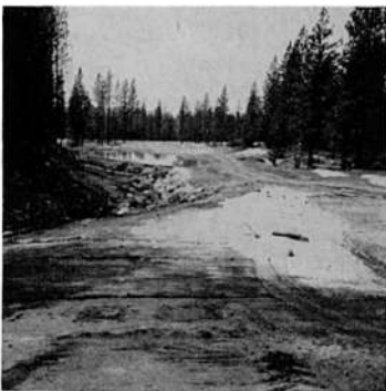
Fairway during construction . . .
