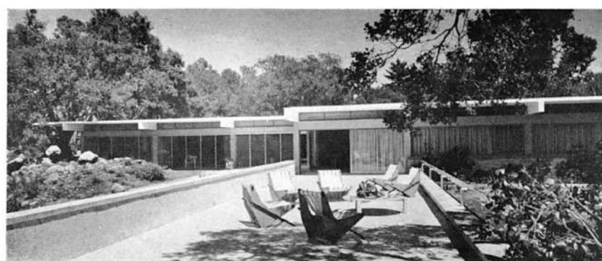
Tremaine House, Santa Barbara, 1948
