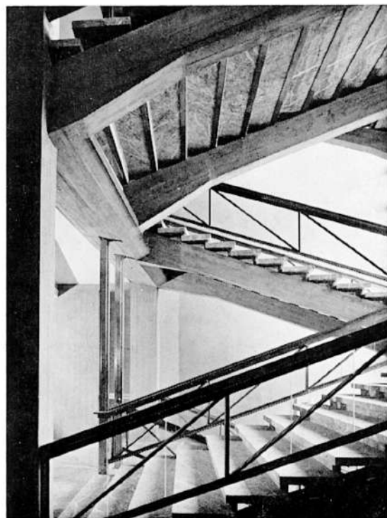
Fior di Pesco Carnico marble stairway, Savings Bank, Florence. Architect Giovanni Michelucci.
