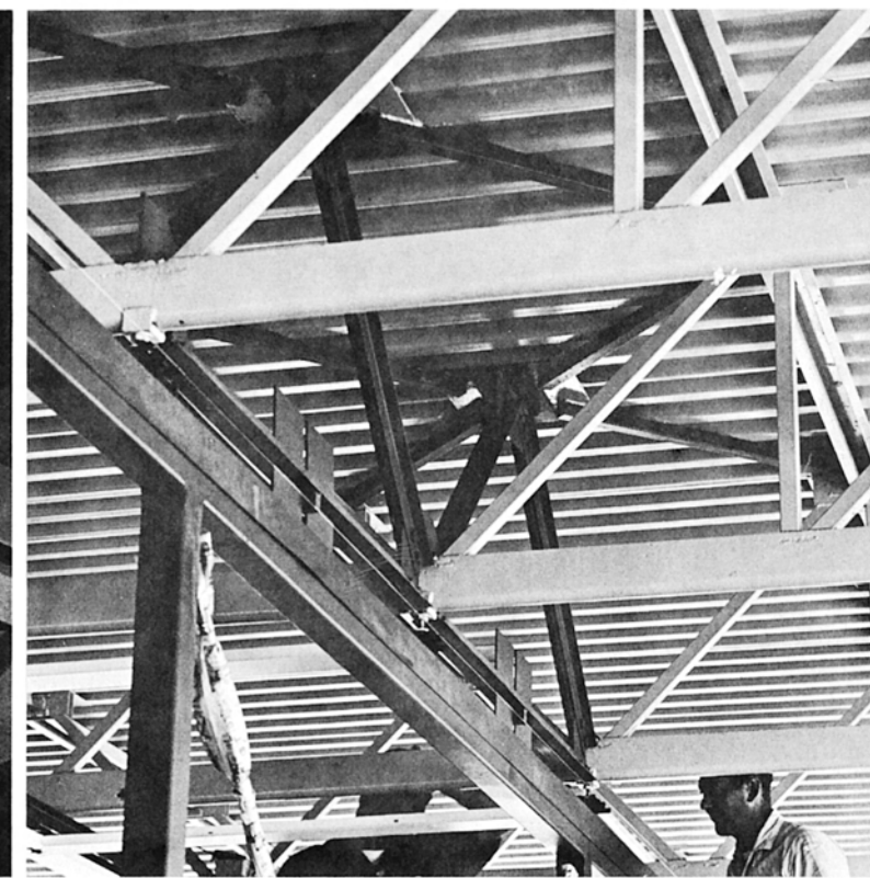
At left, hinged truss-decks are in place but still folded. After unfolding, the 10'-wide decks are welded to adjoining sections. Center left, workmen are installing lighting coffers which go into 3' sandwich between roof deck and ceiling (center right and drawing on page 16) which also carries all service ducts.
