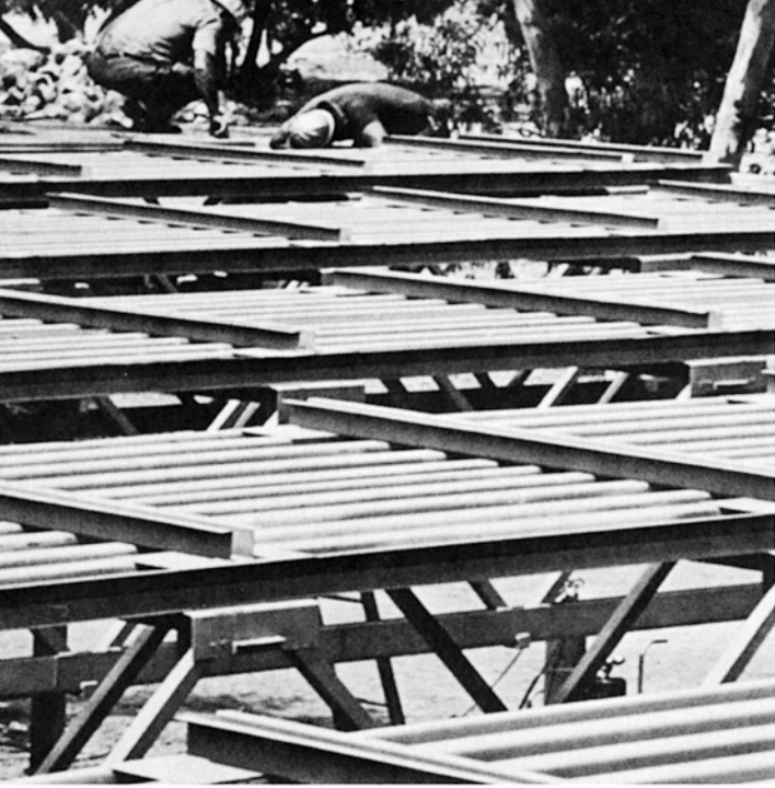
At left, hinged truss-decks are in place but still folded. After unfolding, the 10'-wide decks are welded to adjoining sections. Center left, workmen are installing lighting coffers which go into 3' sandwich between roof deck and ceiling (center right and drawing on page 16) which also carries all service ducts.
