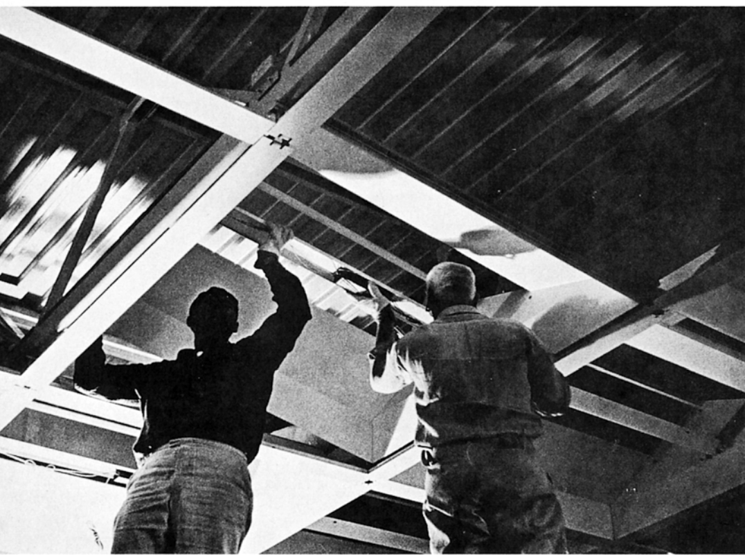
At left, hinged truss-decks are in place but still folded. After unfolding, the 10'-wide decks are welded to adjoining sections. Center left, workmen are installing lighting coffers which go into 3' sandwich between roof deck and ceiling (center right and drawing on page 16) which also carries all service ducts.
