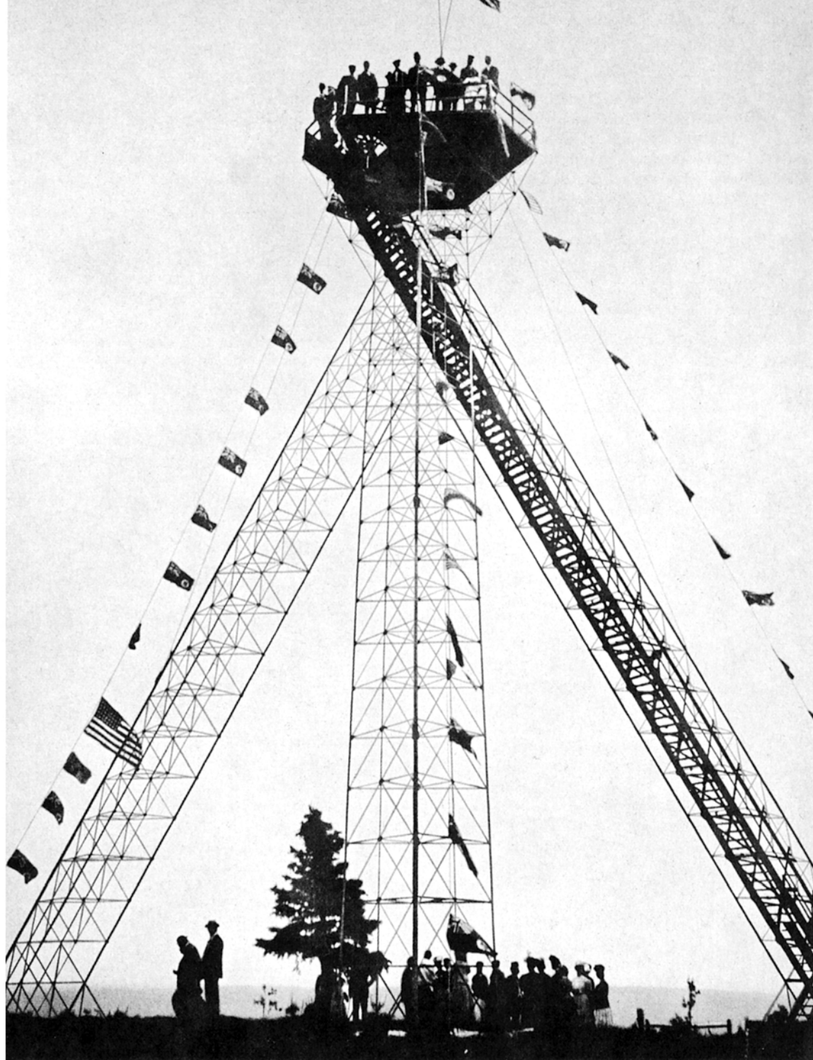
80-foot high space frame tower designed by Alexander Graham Bell and built in 1907. Assembly required 10 days. Photo by John A. D. McCurdy, © Bell Family. Below is the $3 million Gyrotron pyramid at EXPO 67 fun zone.
